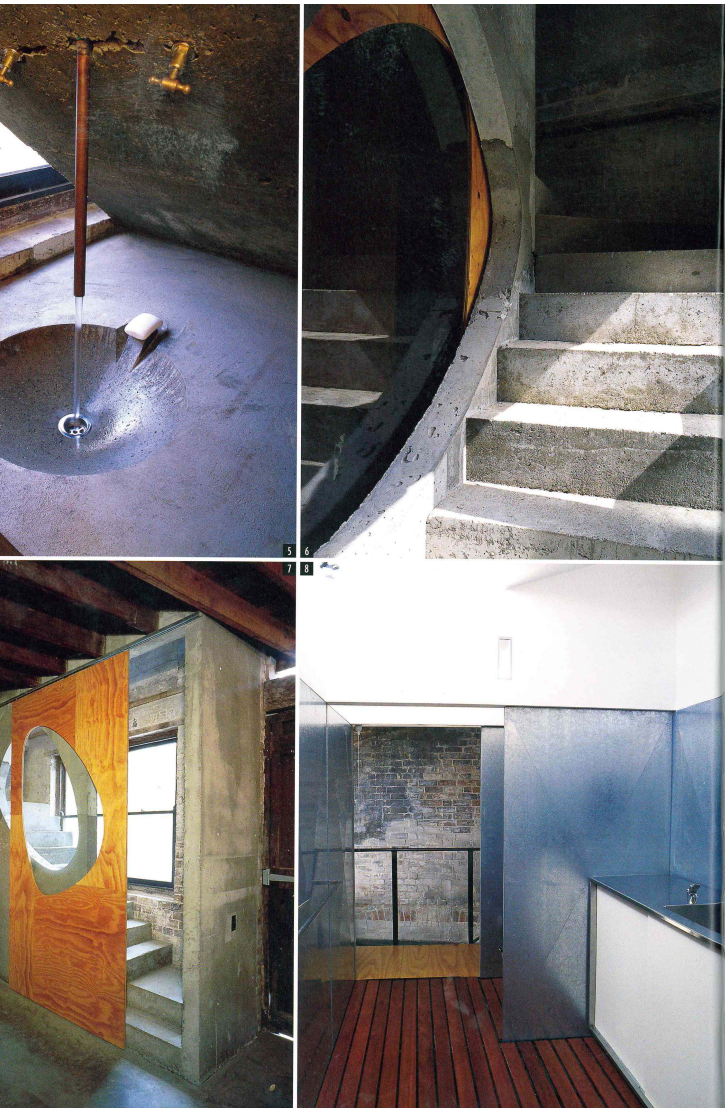
5. Beneath the stairs is a toilet and hand basin formed in concrete. The architect used a wok as the mould for the sink. The water drops from a length of copper pipe. 6. Built in off-form concrete by Drew Heath, the stairs were left rough in keeping with the warehouse's rugged industrial past. 7. A sliding plywood panel screens the concrete stairs. 8. The bathroom bench houses the washing machine and dryer behind sliding colourback glass. The ceiling is lit by the architect's one indulgence: Kreon uplights.
